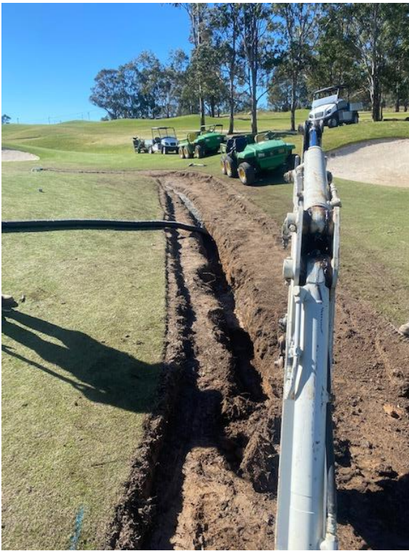
The new drainage line in front of green
